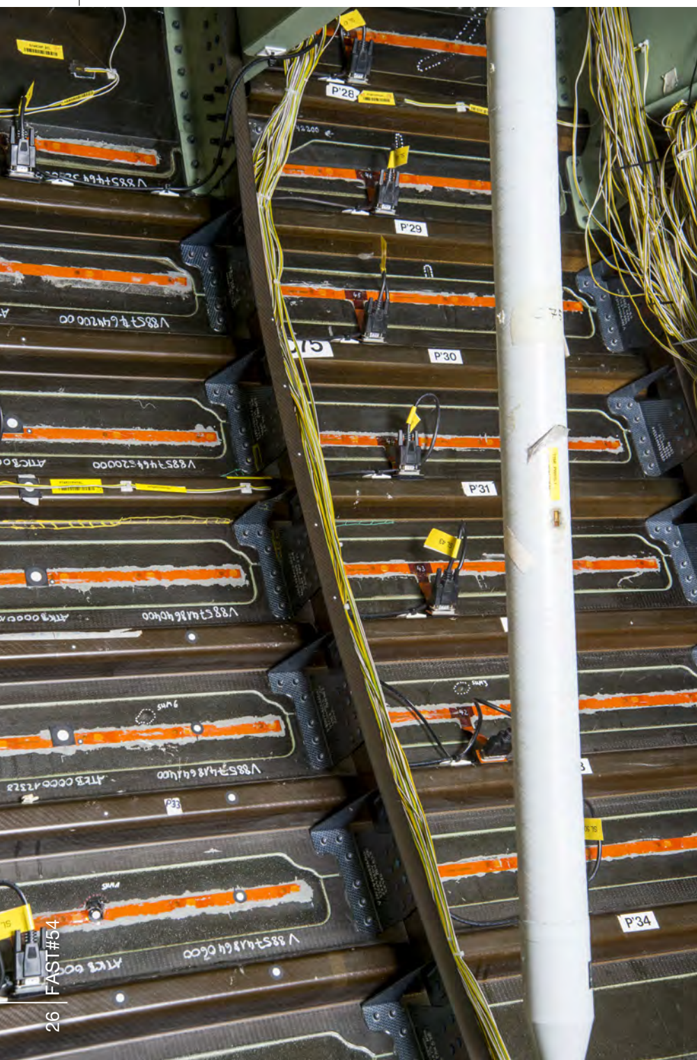
Figures 5 & 6: SHM impact damage detection system sensor network installed in the A350 XWB CFRP composite panel demonstrator of the A340 MSN001.
