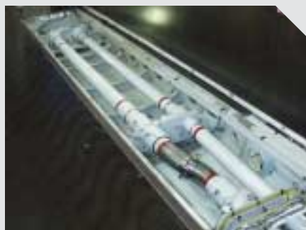
ACT fuel pipes installations
