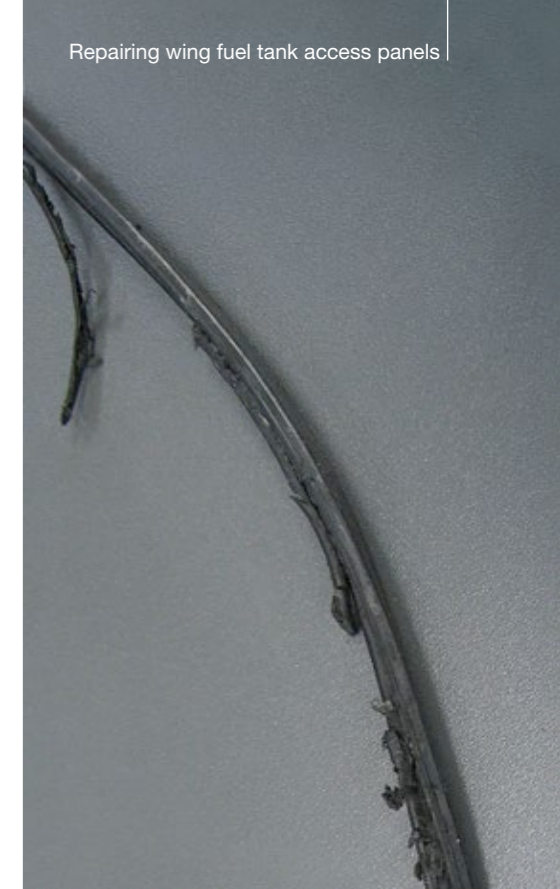
Example of seal fatigue
